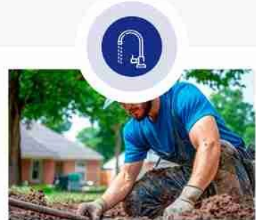
Water Line Repair
