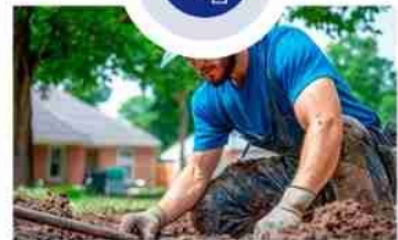
Water Line Repair
