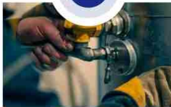
Gas Line Services
