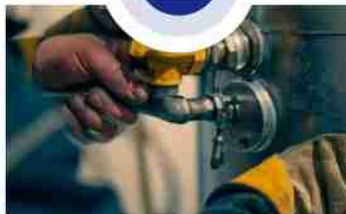
Gas Line Services
