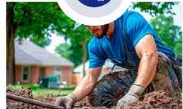
Water Line Repair
